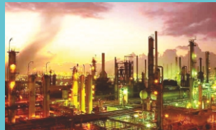
Oil refinery plant
