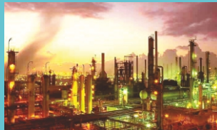
Oil refinery plant
