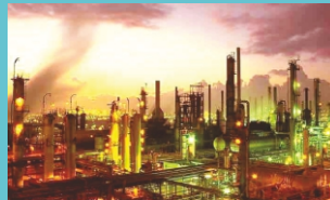
Oil refinery plant
